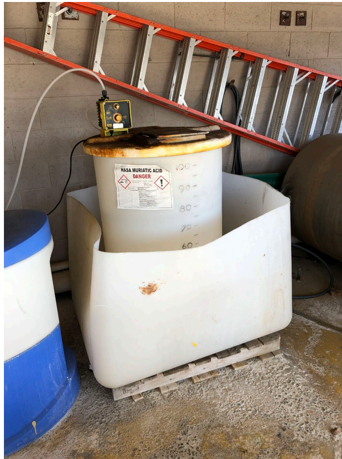
Acid System in Mechanical Enclosure
