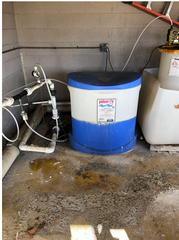
Chlorine System in Mechanical Enclosure
