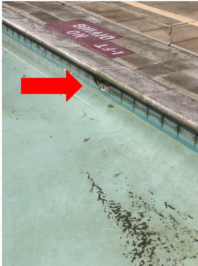
Chipped / Missing Swimming Pool Waterline Tile
