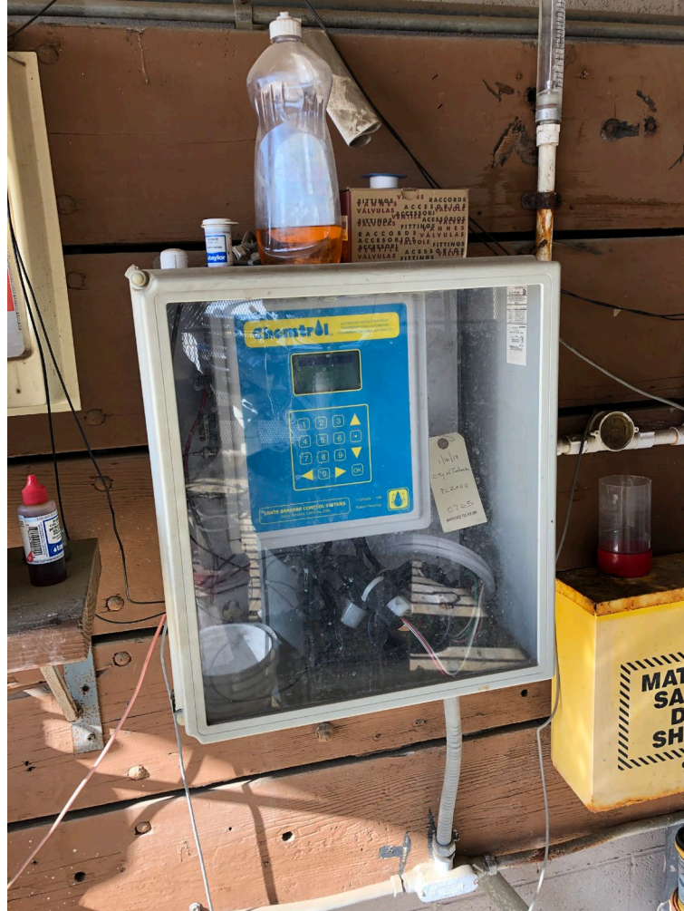
Swimming Pool Chemical Controller
